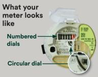
Your meter will look like the one in the diagram above. It might be tricky to read, a top tip take a torch. First lift the opaque cover. There are two key indicators to identify if a meter is registering consumption:
