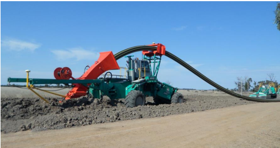
Figure A4 - 2 Pipe plough installing HDPE Pipe
