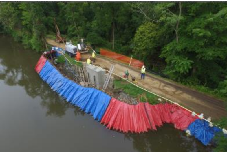
Figure A4 - 4 Portadam Cofferdam for Outfall Construction (Source: Portadam)
