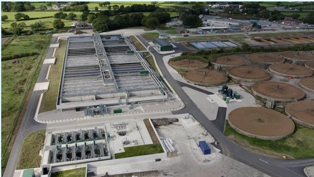
Figure 18: Europe's largest new build Nereda® solution at Blackburn WwTW
